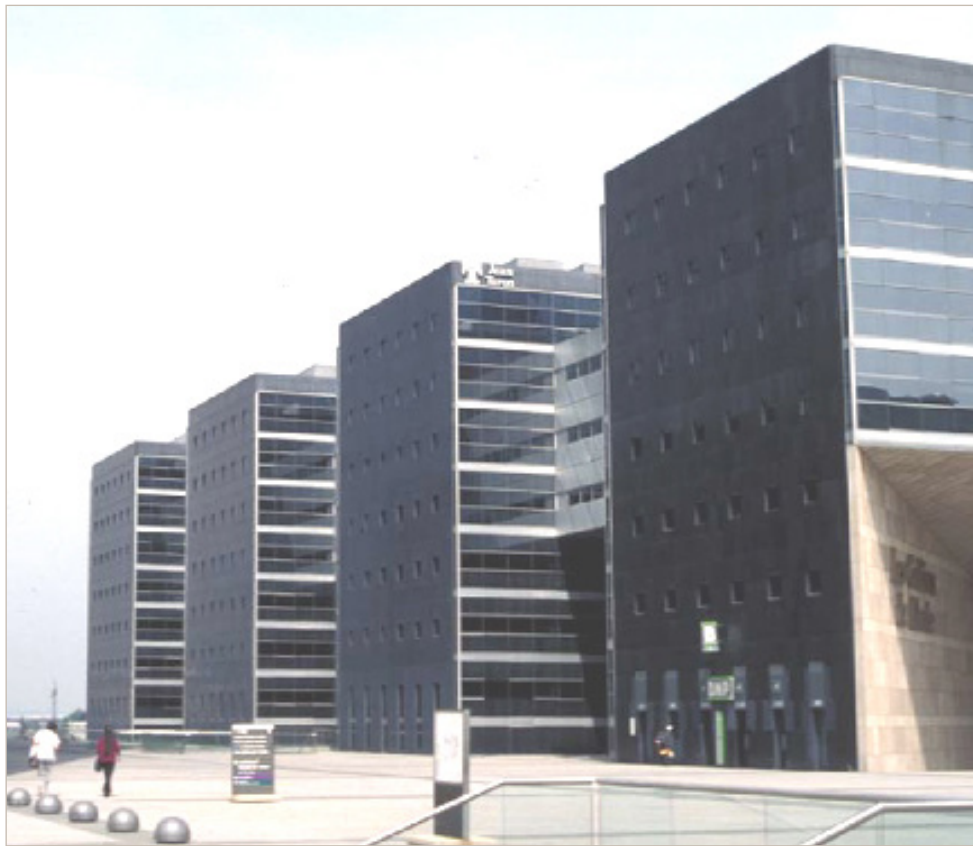
Very separate office buildings in La Defense near Paris. Photo David Kolb
