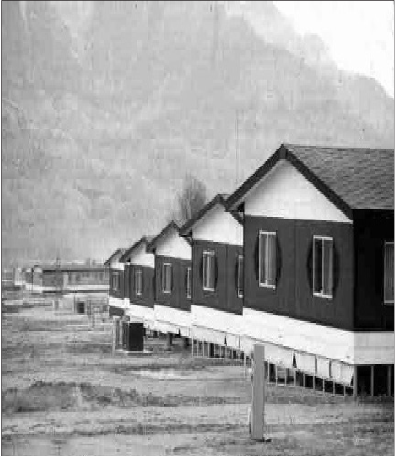
Housing built for a mining town in Colorado. There is no roughness in the sense discussed here. The houses are designed elsewhere and plopped down without reference to each other or the site. Photo by Eric Magolis
