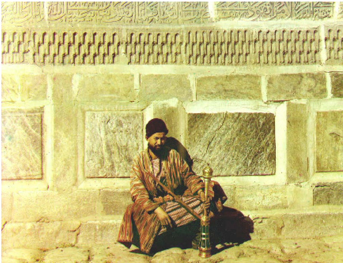
A stone wall in Central Asia built with large blocks at the bottom and a continuing gradient of smaller stones and carved motifs as it moves upwards.
